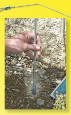
1. Choose location to insert EARTH ANCHOR. Insert Pounding Rod into anchor and pound stake in. Apply a drop of oil or spray some silicone in the hole to aid in removal of the rod. Twisting the rod also aids in the rod removal.
